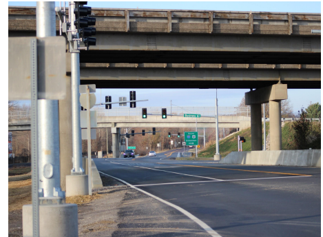
MODOT construction includes new traffic stop lights with crosswalks and sidewalks.
