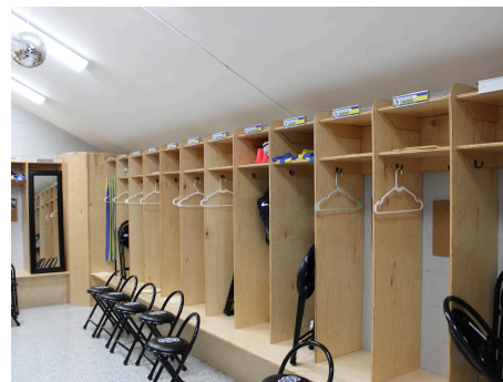
Newly renovated girls locker room.
